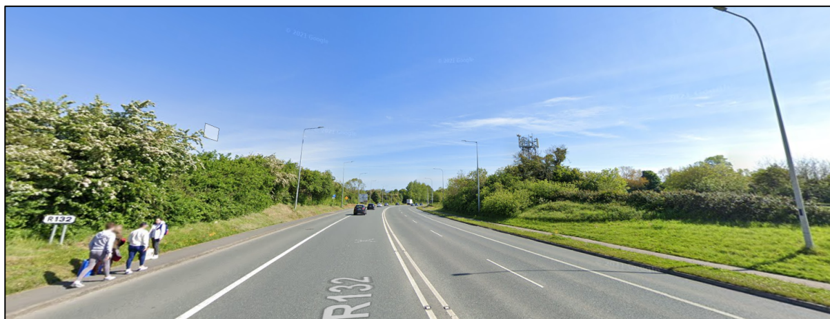
Figure 14: Dublin Road / R132 Without Crossing Facilities
